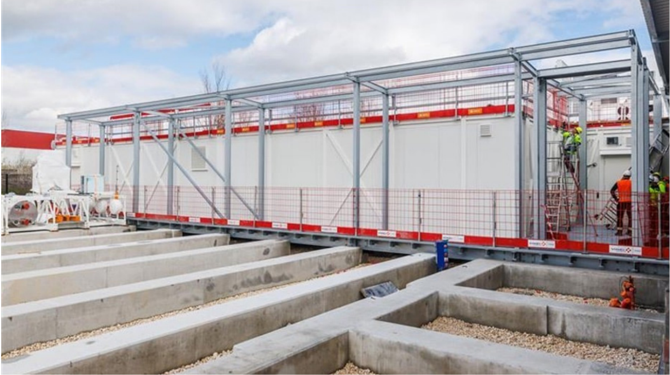
Modular Data Center Under Construction Source: Equinex
